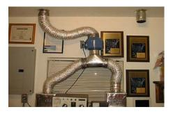
Now that I know it all works, the fan is mounted in the attic and only two drops of ductwork come down from the ceiling to the 6" x 6" pickup plenum (see Photos below) sitting on the amp exhaust. (Your local HVAC supplier can make you a duct board plenum.)
