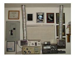
I have the remote variable speed control mounted by my operating position and it works like a dream. After taking temperature readings at the amp exhaust, use of the exhaust system has dropped the temperature down from 150° to less than 120°. This can only make the tubes happy! Also, my air conditioning system can now hold the room at a nice 75° even when it's 95° + outside.
